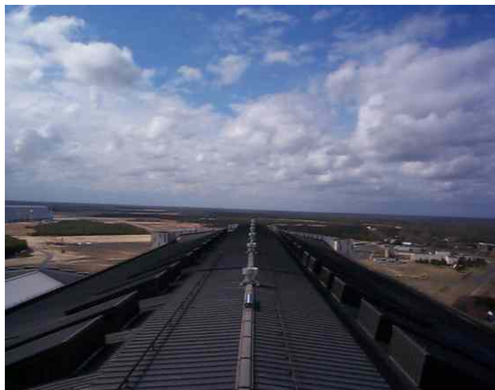
Hanger One from top of Hanger One. Photo by WX2NJ
